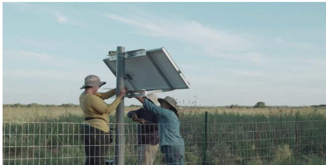
Seismometers like this one help track earthquakes across Texas as part of the TexNet Seismic Monitoring Network.
